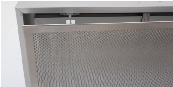
Photo 1: Friction catches hold the outer screen to the fan module housing.
